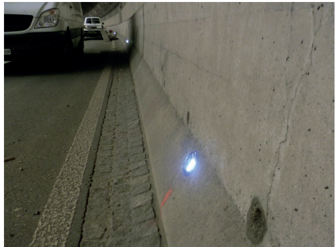
Tunnel Stephanshorn St. Gall
